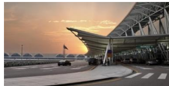
The New Guangzhou Baiyun Airport T2 Year of completion : 2018 Annual passenger handling capacity: 45 million
