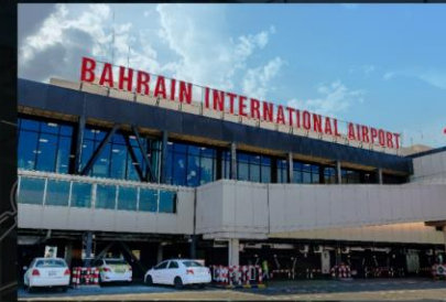
(August) - Handover and demolishing works of Phase 2
